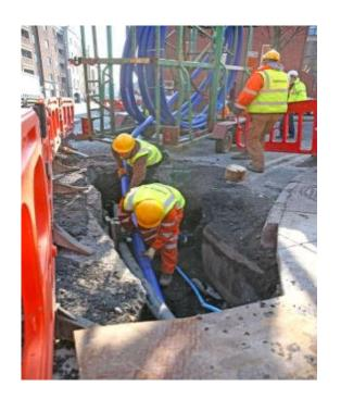
Where technically possible, the replacement of public water mains will be carried out using innovative technology and trenchless methods of pipe replacement. This will help to reduce the number of supply interruptions to customers and will also minimise the level of disruption on local roads. We understand that there will be some level of disruption to customers but we will endeavour to keep this to a minimum.
